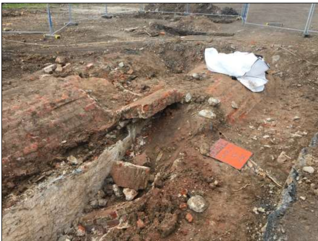
Plate 68. Interface of Gallery 2 with Gallery 3, showing the southern side wall of Gallery 2 extending under the span of the elliptical vaulted roof of Gallery 3.
