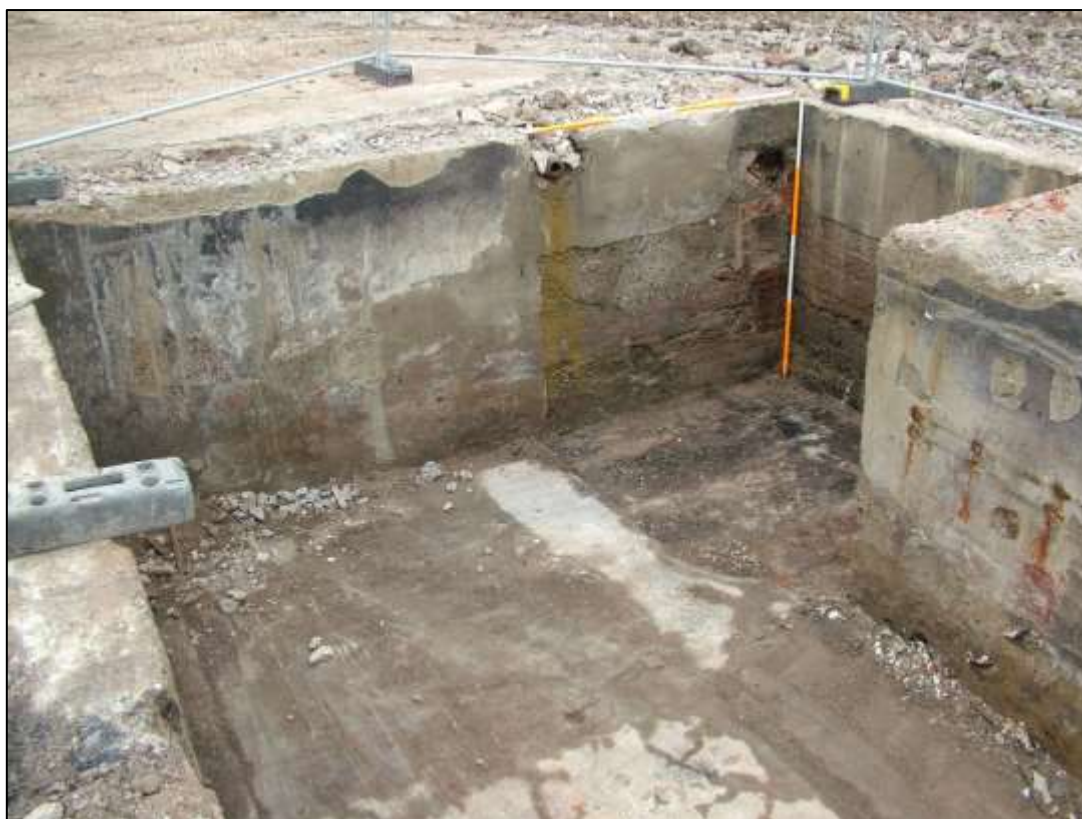
Plate 11. Area 2 – Basement of Temporary No 4 / Block 9 looking NW
