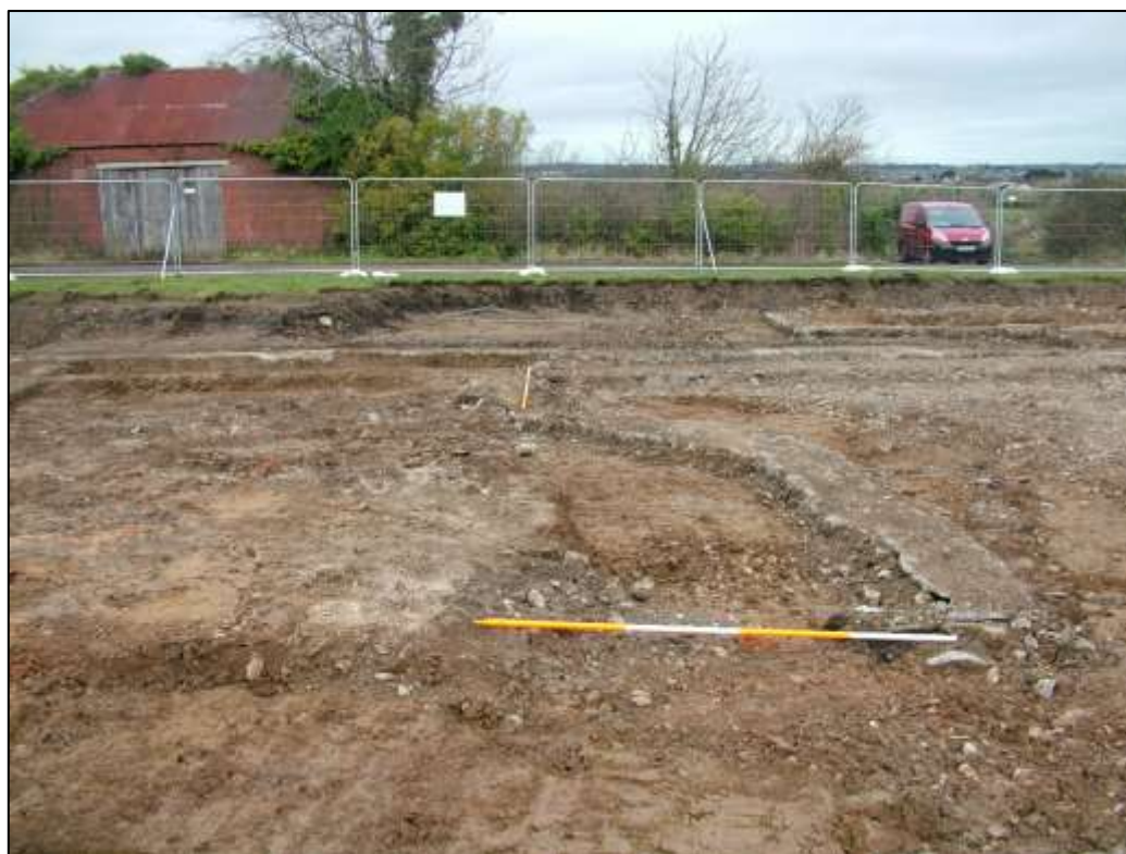
Plate 25. Area 1 – Curving wall, part of original gateway to Portrane House yards looking N
