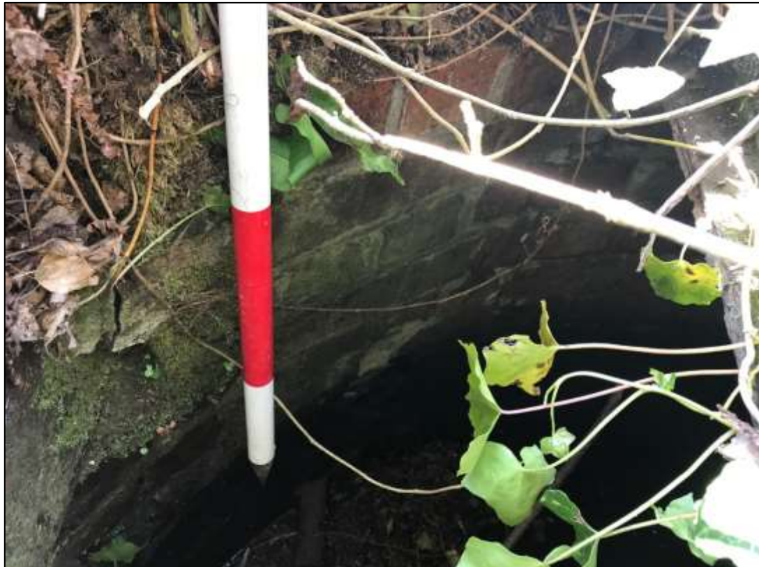
Brick lined well
