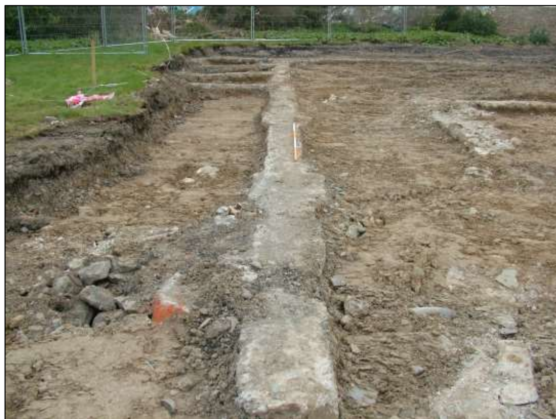
Plate 32. Area 1 – Temporary No 2 / Block 8/8a, dormitory, eastern foundation looking S to storage annex
