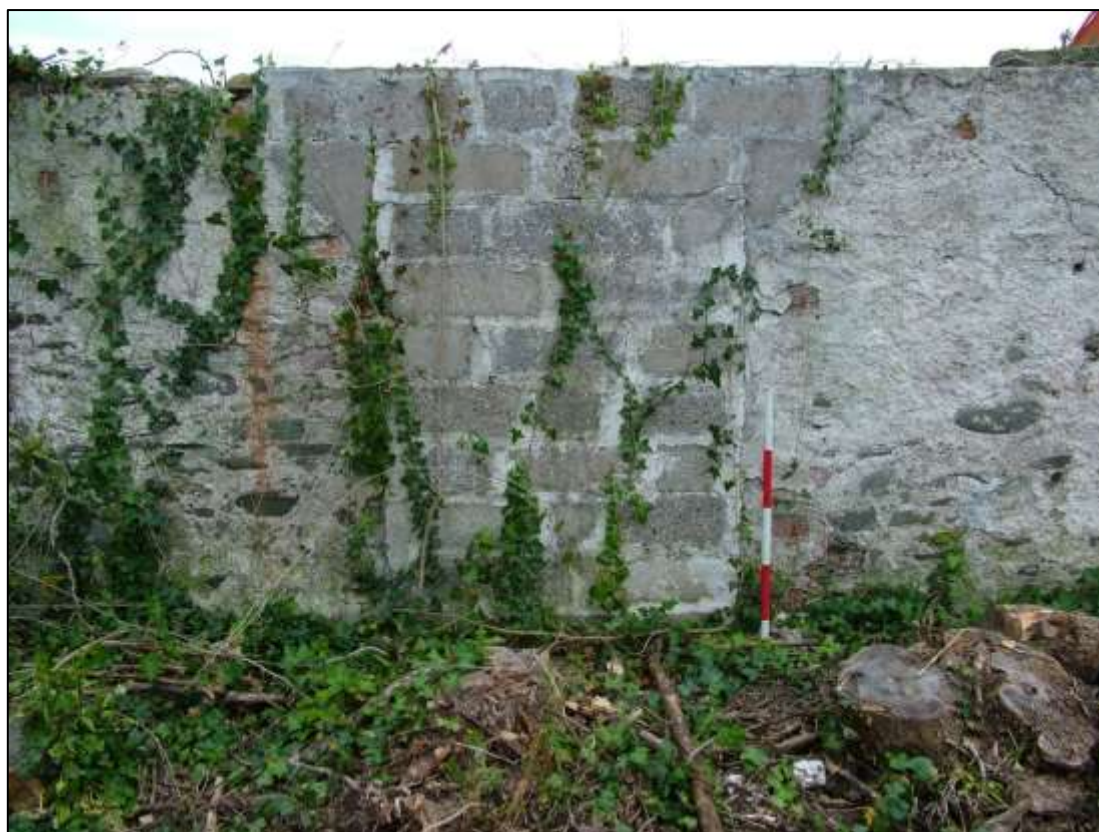
Plate 54. Wall 2 (Main Wall) west facing elevation
