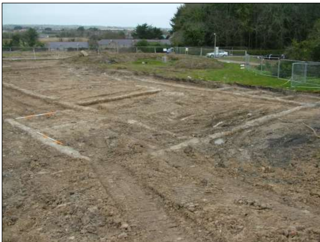
Plate 29. Area 1 – Temporary No 2 / Block 8/8a, eastern dormitory foundation looking NE
