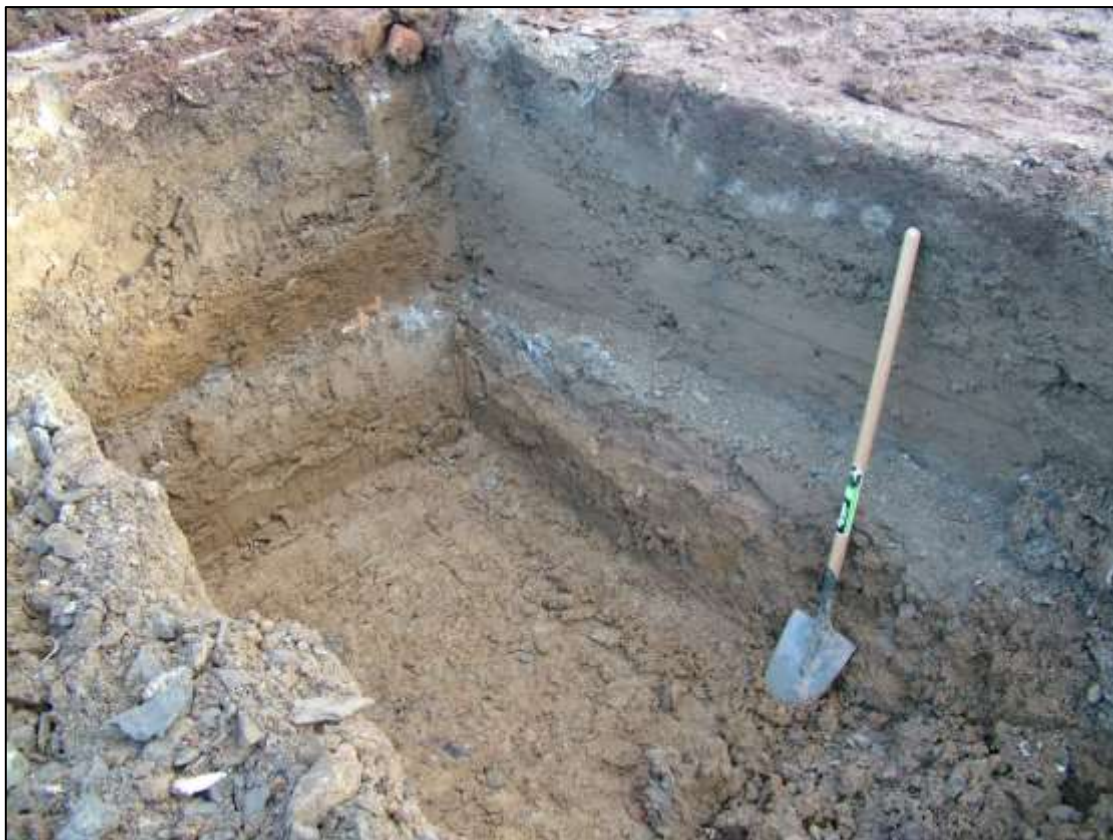
Plate 18. Area 2 – Temporary No 3 / Block 11, depth of foundation. Looking NE
