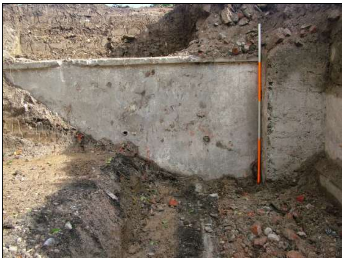
Plate 42. Area 3 – Portrane House, basement level exterior. Retaining wall, c. 1937.
