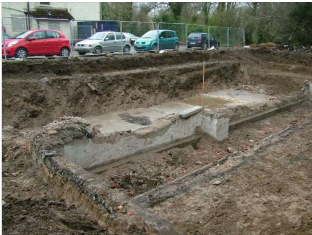
Plate 45. Area 3 - Portrane House, basement level. Looking SW
