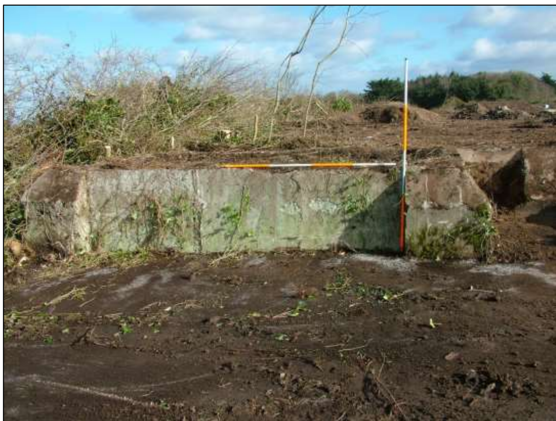
Plate 7. Area 2 – Extant foundation of Temporary No 4 / Block 9. NW corner looking E
