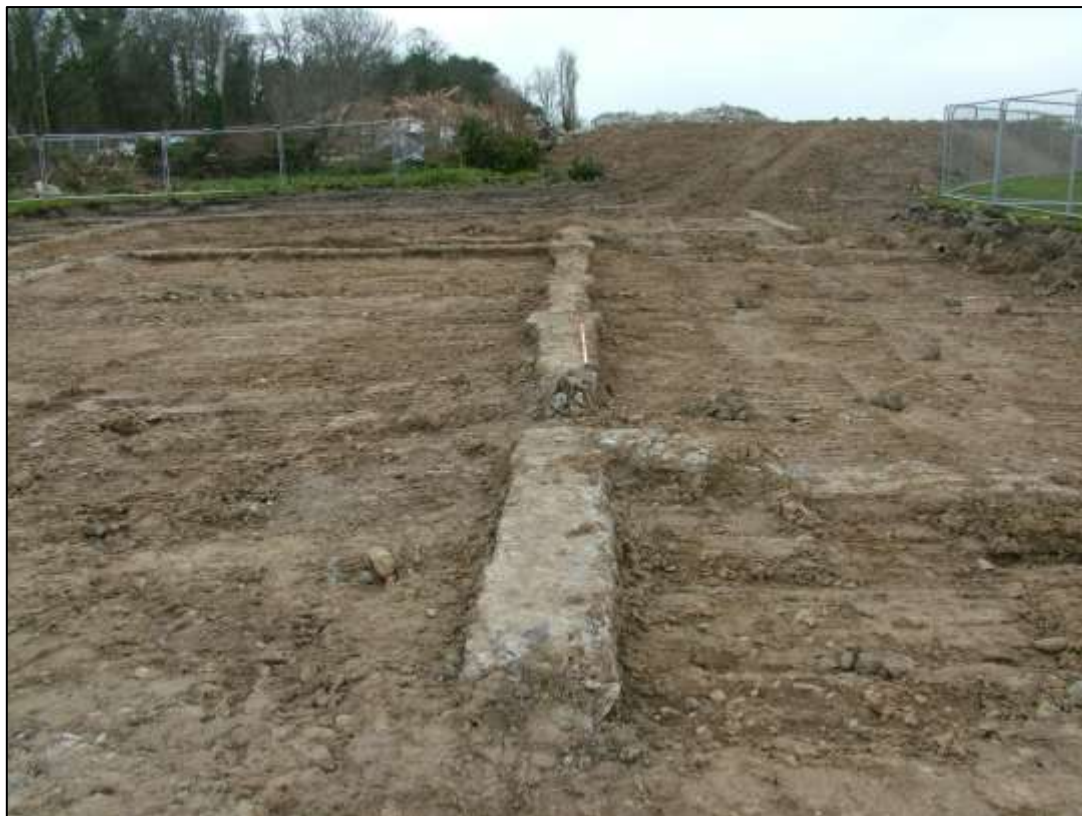
Plate 33. Area 1 – Temporary No 2 / Block 8/8a, dormitory, western foundation looking S to storage annex
