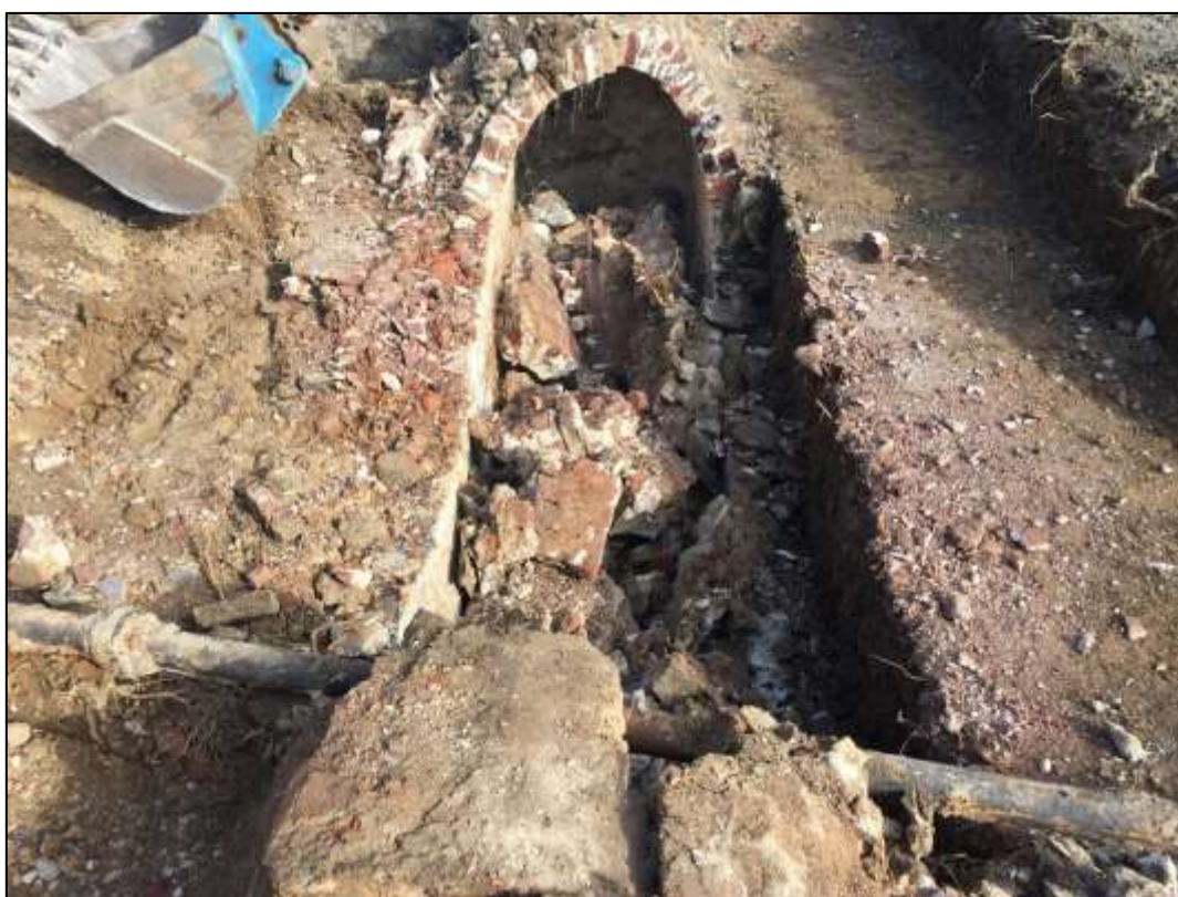
Plate 67. Gallery 1 / 2 during demolition. Looking E.
