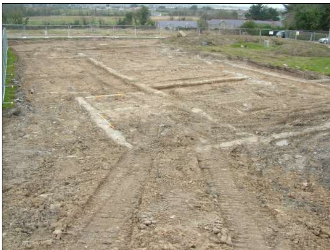
Plate 30. Area 1 – Temporary No 2 / Block 8/8a, eastern dormitory foundation looking N
