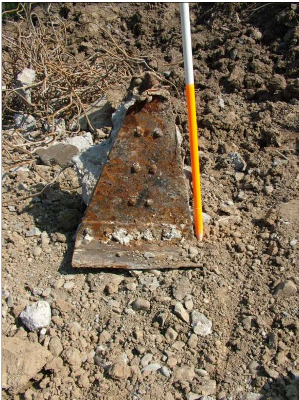
Plate 13. Detail of cast iron footing Temporary No 4 / Block 9
