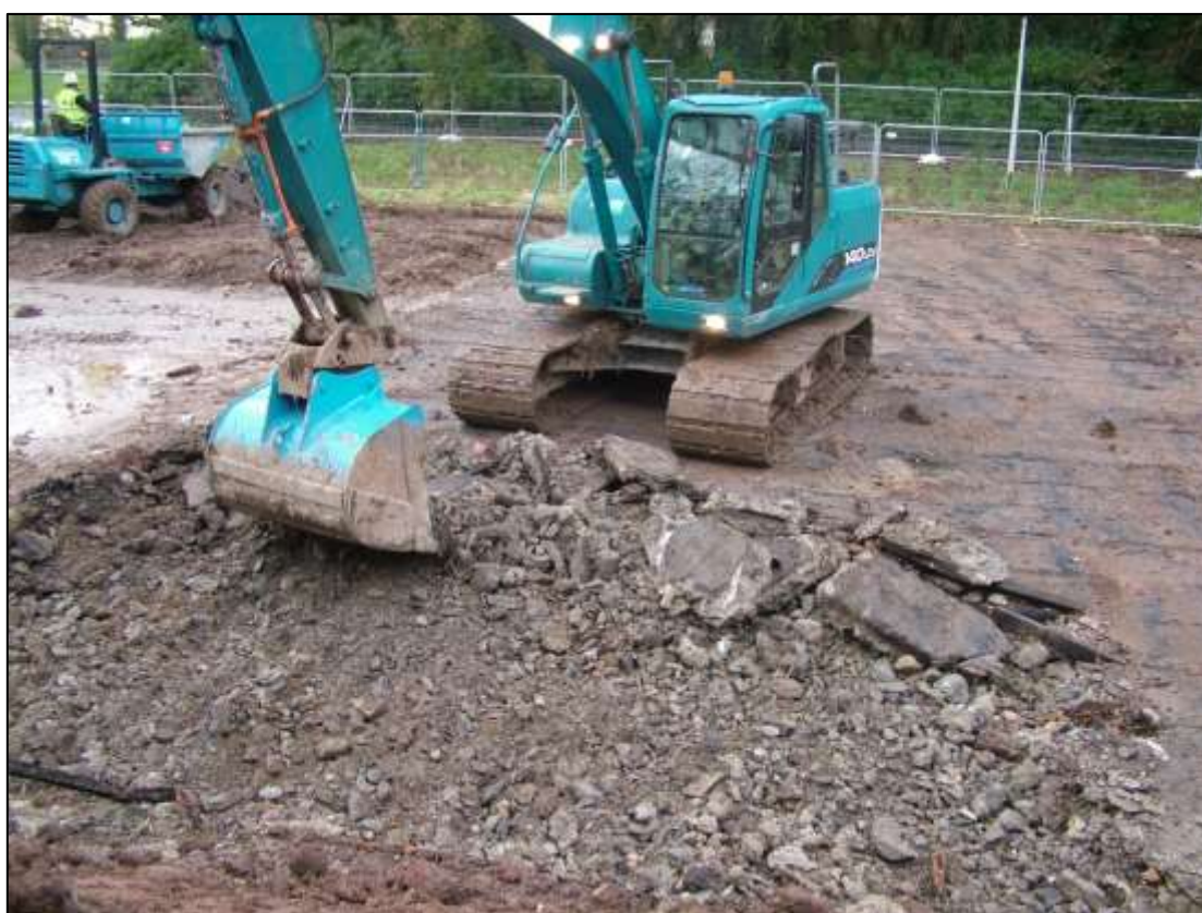
Plate 17. Area 2 – removal of asphalt subfloor, Temporary No 3 / Block 11. Looking S
