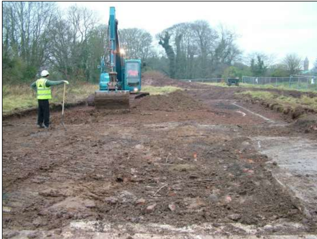
Plate 5. Area 2 - Stripping topsoil from Temporary No 4 / Block 9 looking east
