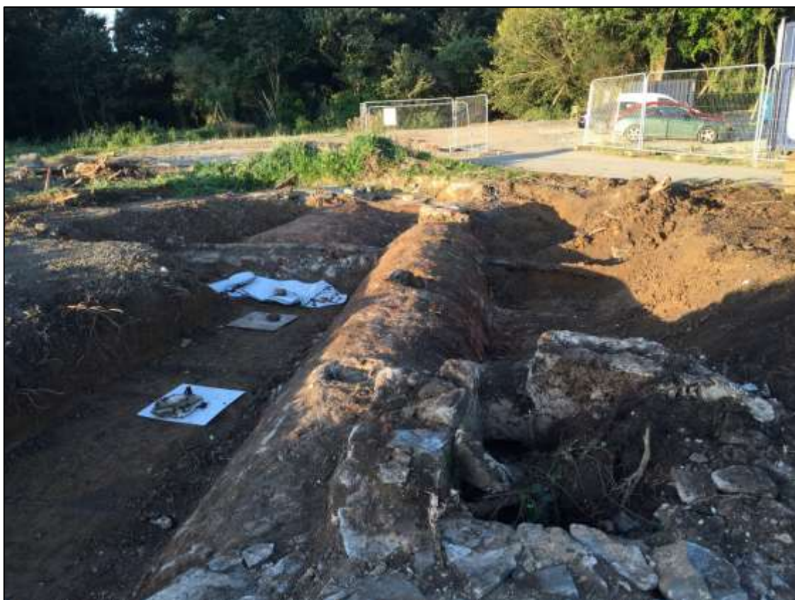
Plate 62. The service tunnel vaulted roof exposed during excavation. Looking W
