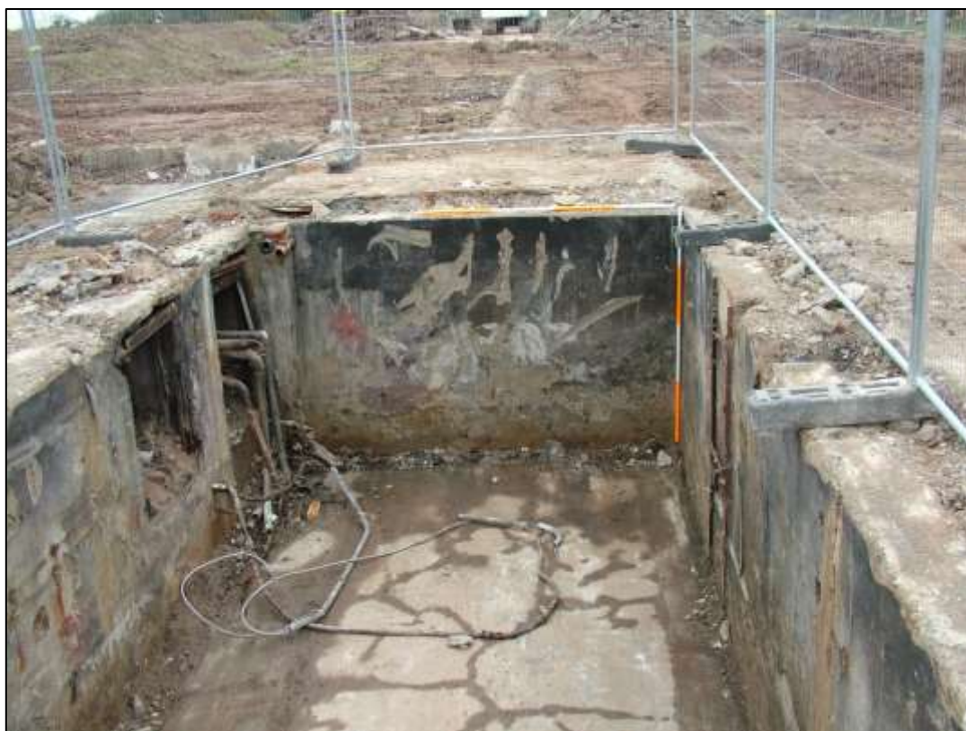
Plate 9. Area 2 – Basement of Temporary No 4 / Block 9 looking east
