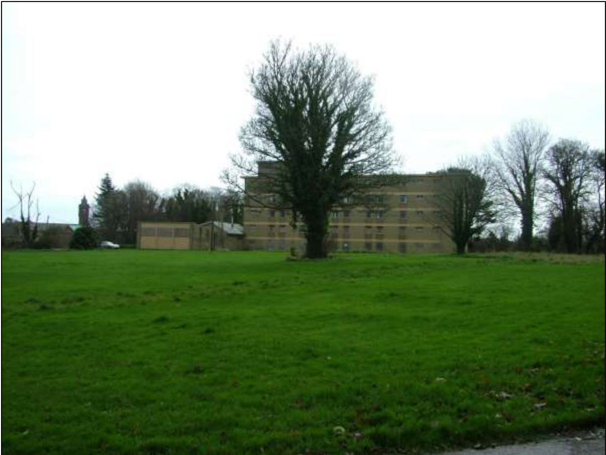
Plate 70. View across Area 1 prior to commencement of site works (December 2015)
