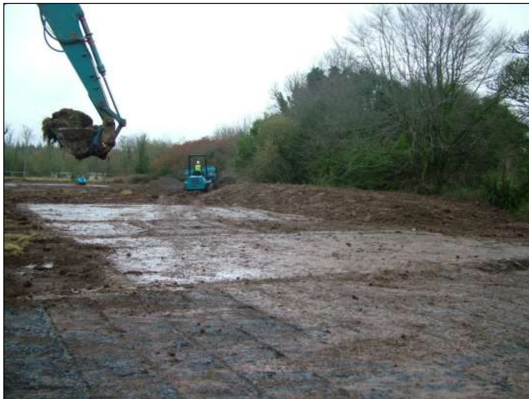
Plate 14. Area 2 – Temporary No 3 / Block 11 during topsoil strip looking NW
