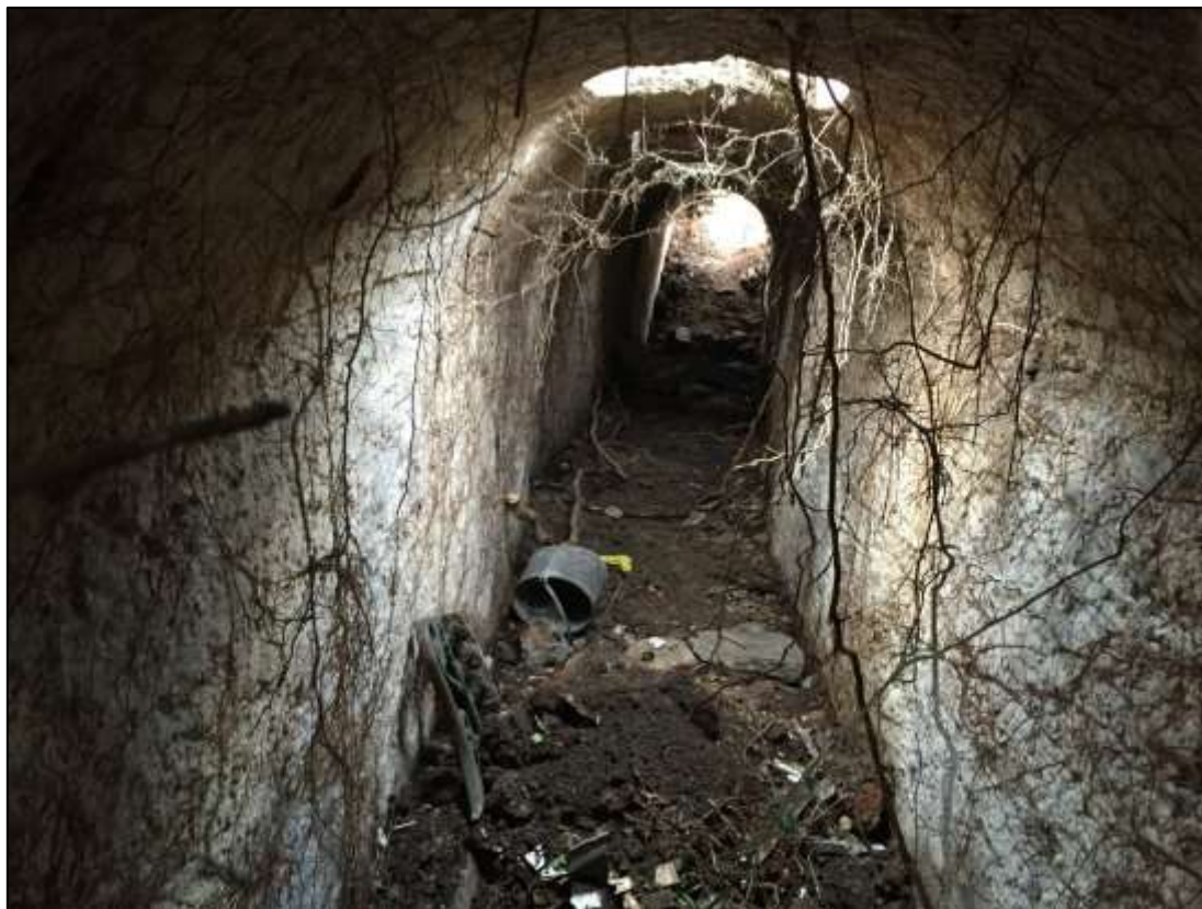
Plate 60. Service tunnels looking E
