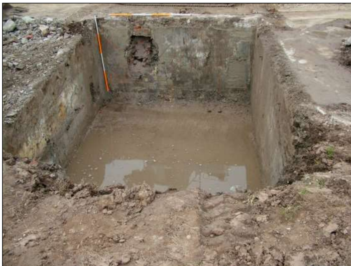
Plate 19. Area 2 – Temporary No 3 / Block 11. Basement. Looking S
