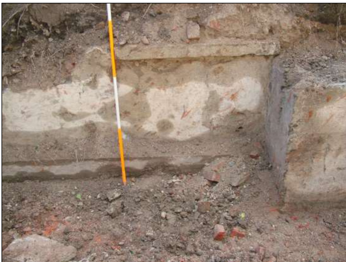
Plate 41. Area 3 – Exterior wall face, basement level, Portrane House. Looking S
