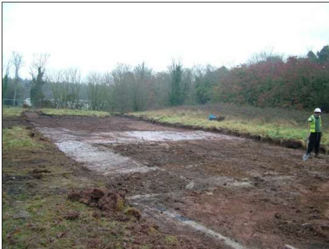
Plate 4. Area 2 – Stripping topsoil from Temporary No 4 / Block 9 looking west
