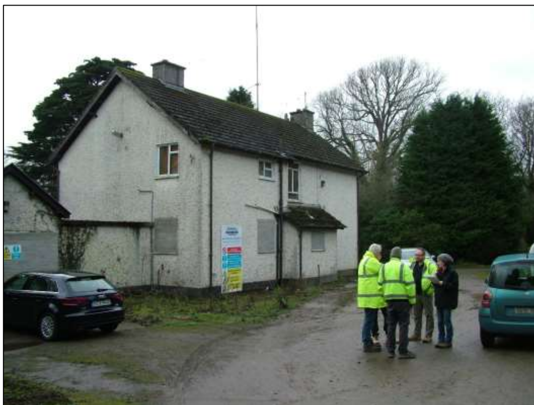
Plate 69. House 100 (1950s-1960s) raised on the site of Portrane House. Looking SW
