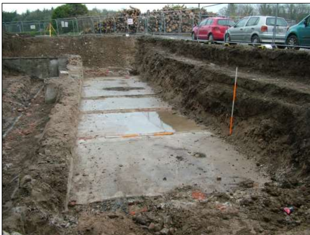
Plate 44. Area 3 – Portrane House, basement level. Looking SE
