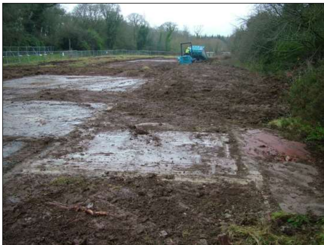
Plate 15. Area 2 – Temporary No 3 / Block 11, toilet annex and main block looking SW
