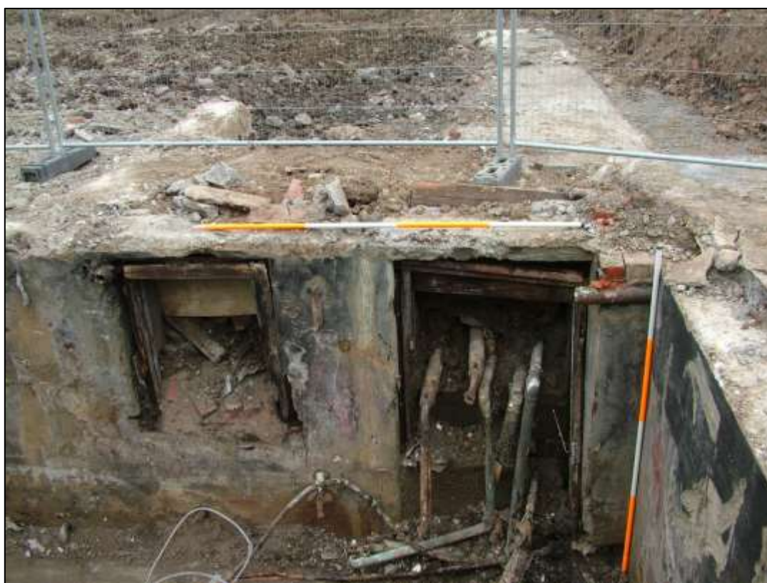
Plate 10. Area 2 – Basement of Temporary No 4 / Block 9 looking north.
