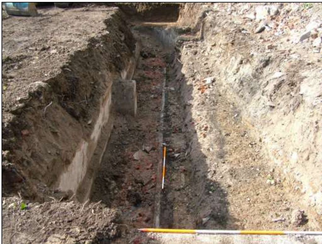
Plate 43. Area 3 – Exterior basement wall Portrane House. Looking W
